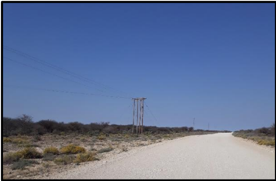
Figure 6. General site conditions
